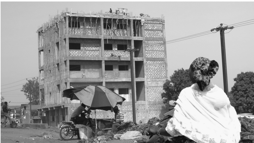
FIGURE 7.3 Commercial building under construction in Bobo-Dioulasso. Photograph courtesy of Souleymane Komboudry
